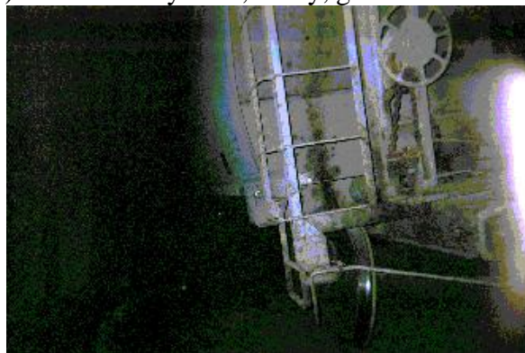
Derailed Cars in Tunnel
