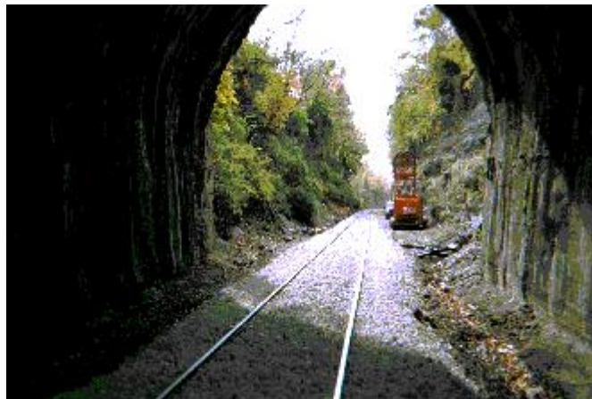
View From Inside Tunnel of MVU
