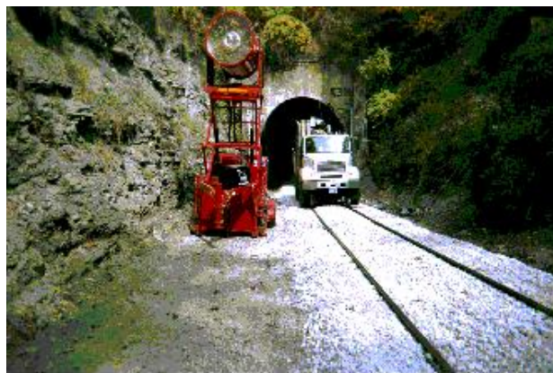
MVU Positioned in Front of Tunnel Portal
