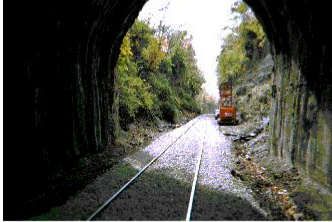
View From Inside Tunnel of MVU
