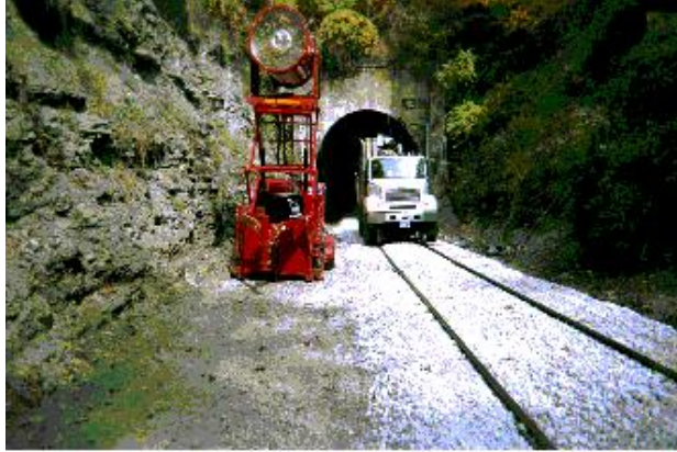
MVU Positioned in Front of Tunnel Portal
